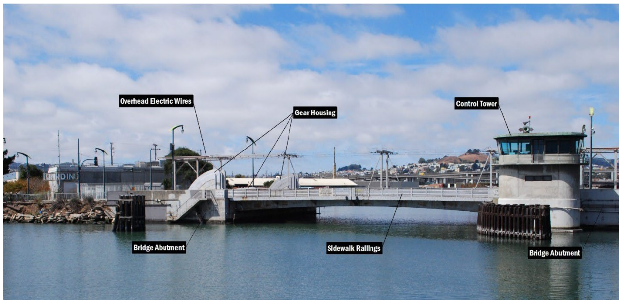
Figure 2.C-1 Islais Creek Bridge East Elevation
