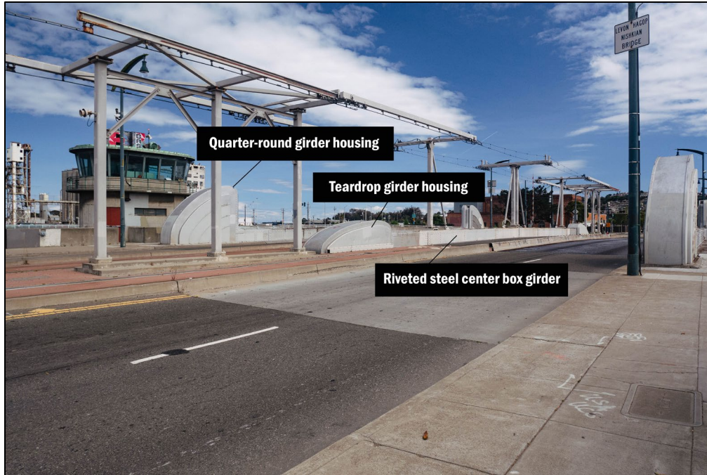
Figure 4.B-1 Above-Deck Character-Defining Features, Facing Southeast
