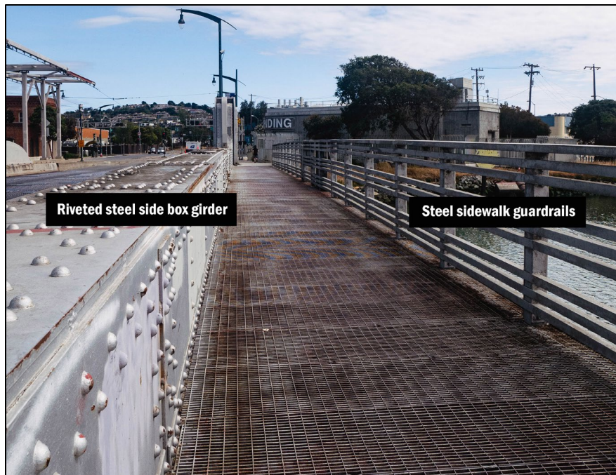
Figure 4.B-2 Above-Deck Character-Defining Features, Facing South
